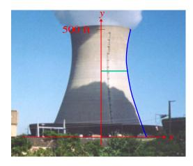
The natural draft cooling tower shown at left is about 500 feet high and its shape can be approximated by the graph of this equation revolved about the y-axis:
